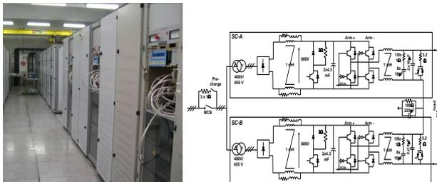
Fig. 7: Example of 4-quadrant power converters used to supply electromagnets.
